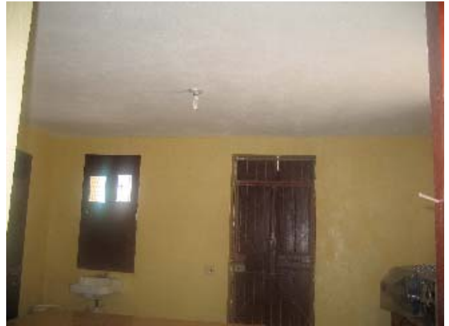
Concrete Roof -- August 2004
